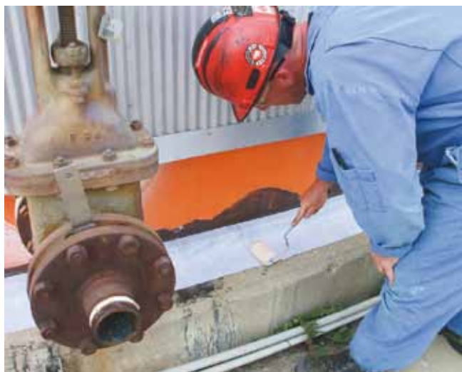
Figure 3. In addition to pipelines, the product is also used for the protection of tank chimes.
