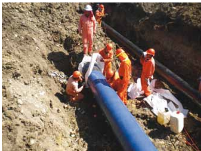
Figure 1. Protection of crude oil pipeline with self-healing coating.
